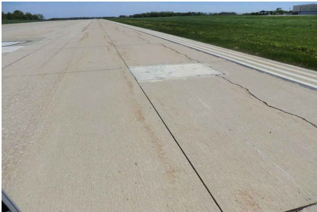
AUM RY1735 001 (LTD Cracking)
